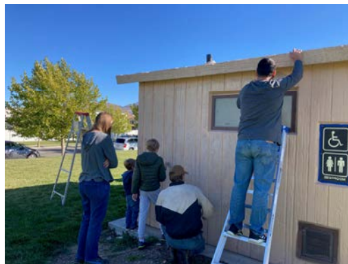
Volunteers Painting the Restrooms at Copper Canyon Park
